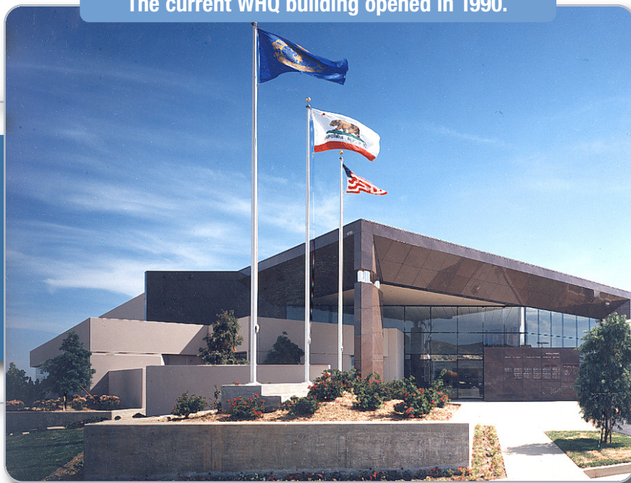
The current WHQ building opened in 1990.
