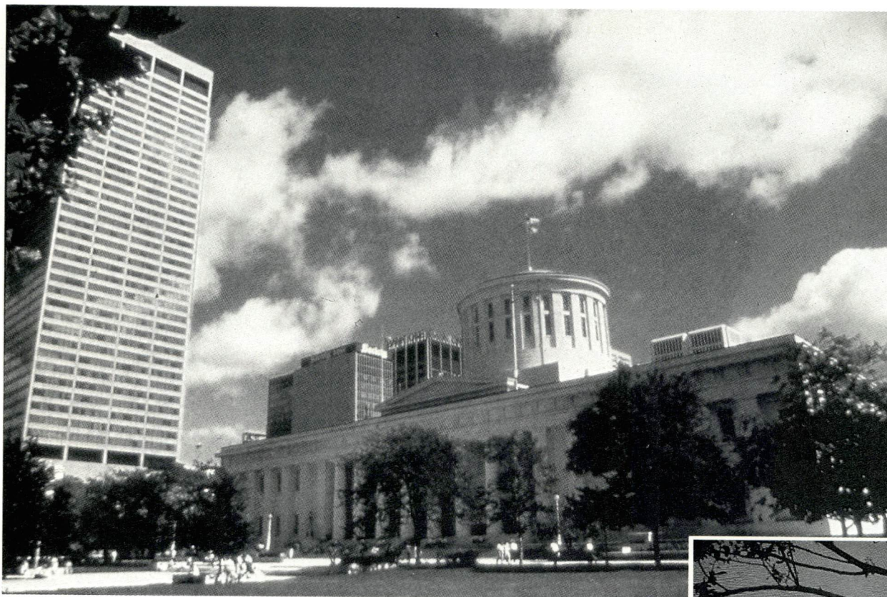
Architectural Contrast—The modern, 41-story State Office Tower soars above the classic, delicate Greek Revival architecture of the State Capitol building.
