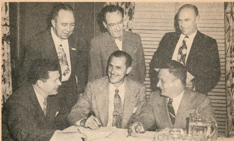
NEARING THE END
